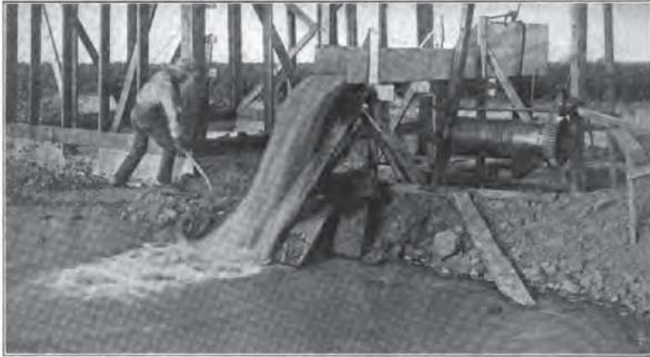
At an average depth of fifty feet, in Madera county, California, an abundance of water is obtained. Electrical energy has solved the cost of pumping problems
